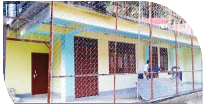
Infrastructure upgradation of school, Sikkim
