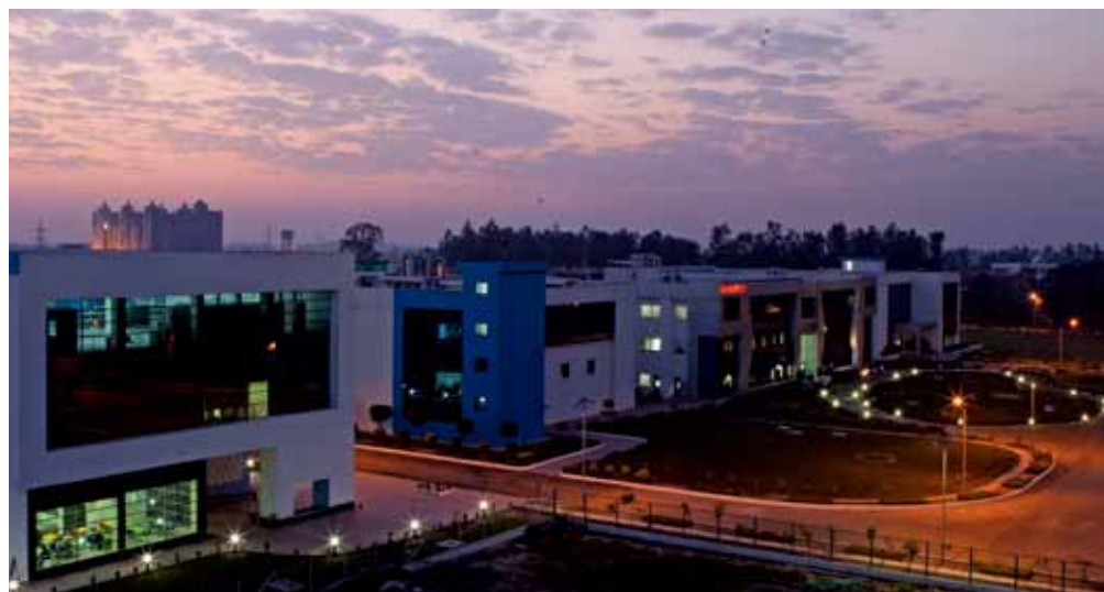
Ranbaxy Plant, Mohali, India
